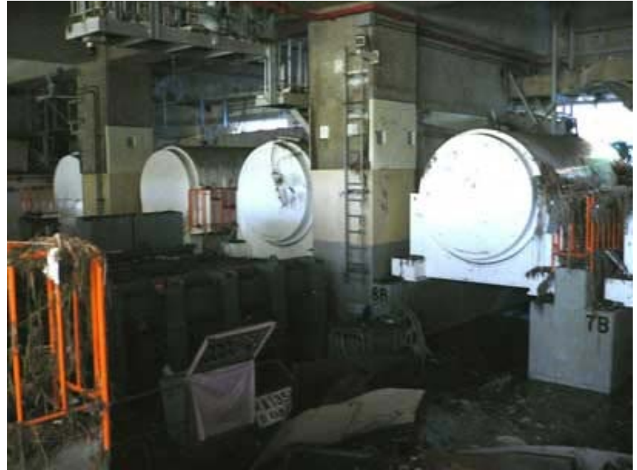
Spent fuel storage casks at Fukushima after the tsunami
