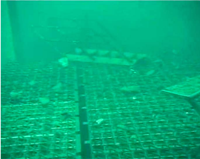
Debris on top of fuel racks in Unit 4 pool
